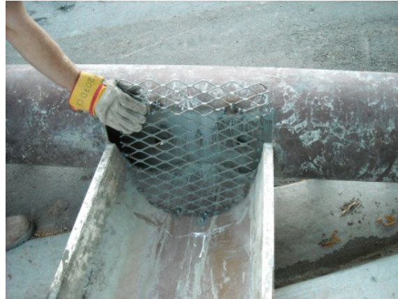
Figure 3: Installing the removable screen.
