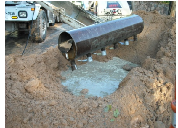
Figure 6: Cleaning the slurry spreader.
