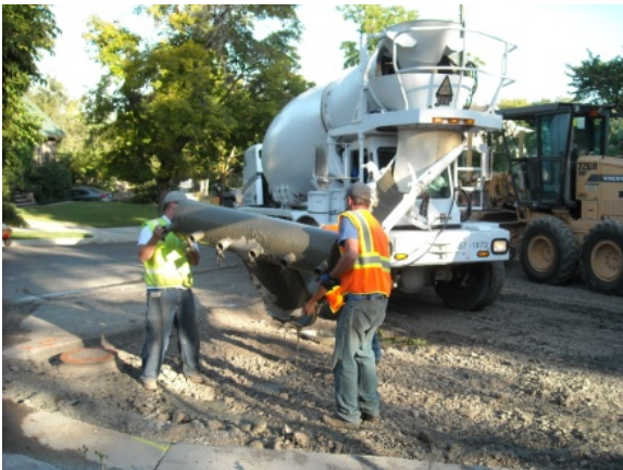
Figure 2: Securing the spreader to a ready-mix truck.
