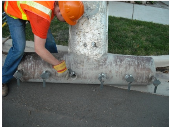
Figure 4: Adjusting the nozzles on the spreader.
