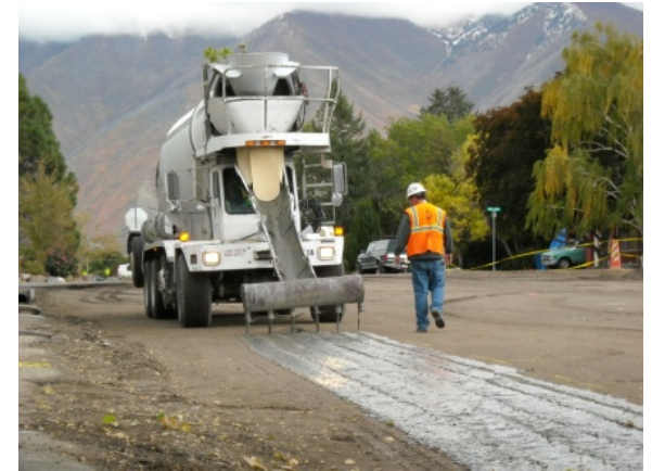
Figure 5: Applying cement slurry with the spreader.
