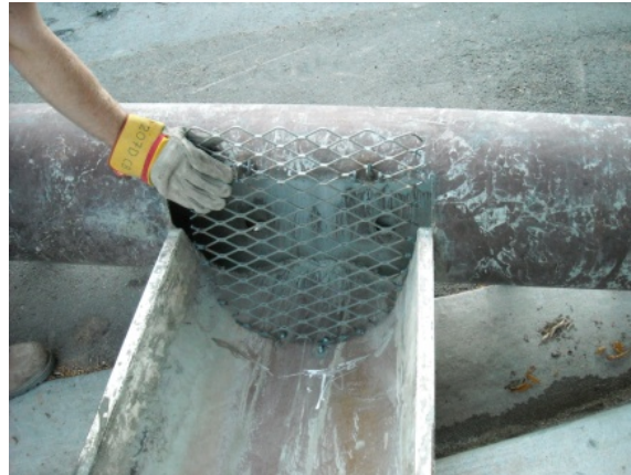
Figure 3: Installing the removable screen.
