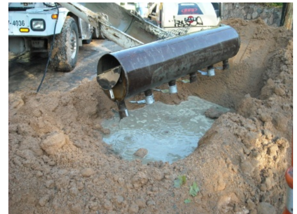
Figure 6: Cleaning the slurry spreader.
