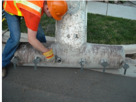
Figure 4: Adjusting the nozzles on the spreader.
