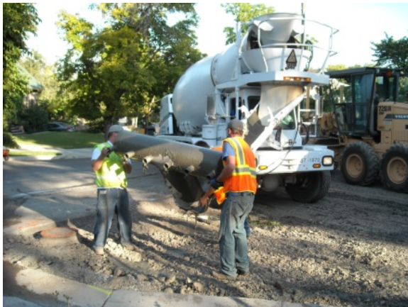
Figure 2: Securing the spreader to a ready-mix truck.
