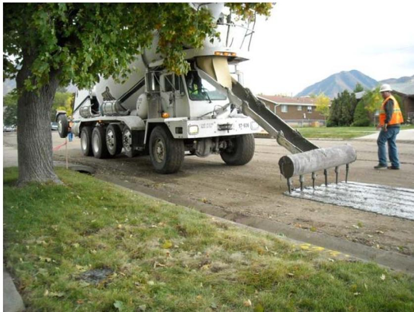
**Figure 1. Application of cement slurry on an urban pavement reconstruction project.**
